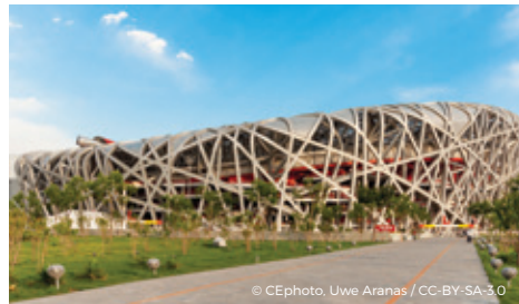
National Stadium, Beijing
